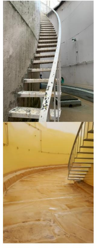
the access ports thru the steel wall had been welded shut. We provided a crane in order to get material and supplies into the containment area. The polyurea material is applied using plural component equipment which have 400 feet of 3 inch hoses. We had to lift the hose section over the high walls in order to seam the pre-sprayed liner material.
